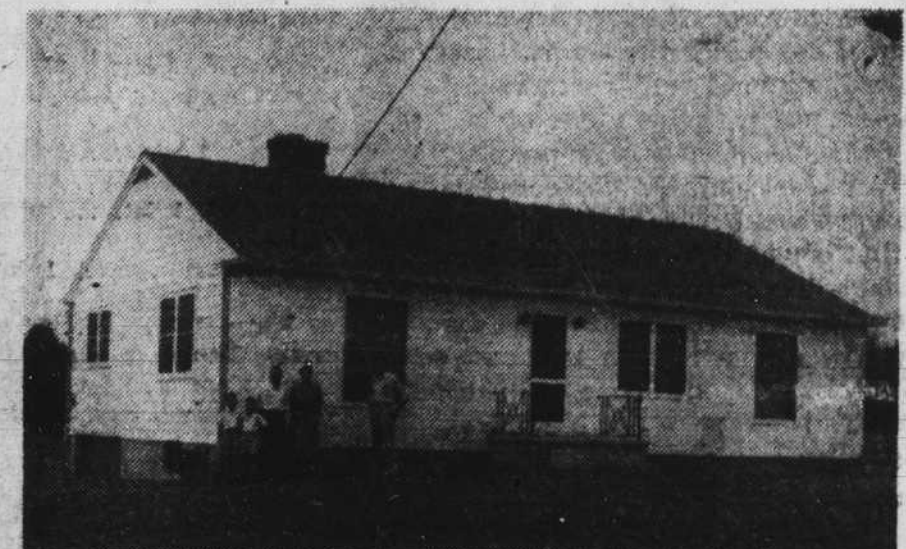
New Home of Mr. and Mrs. Larry S. Coleman of Route 1, Hurdle Mills which was made possible by a loan through the Farmers Home Administration.
