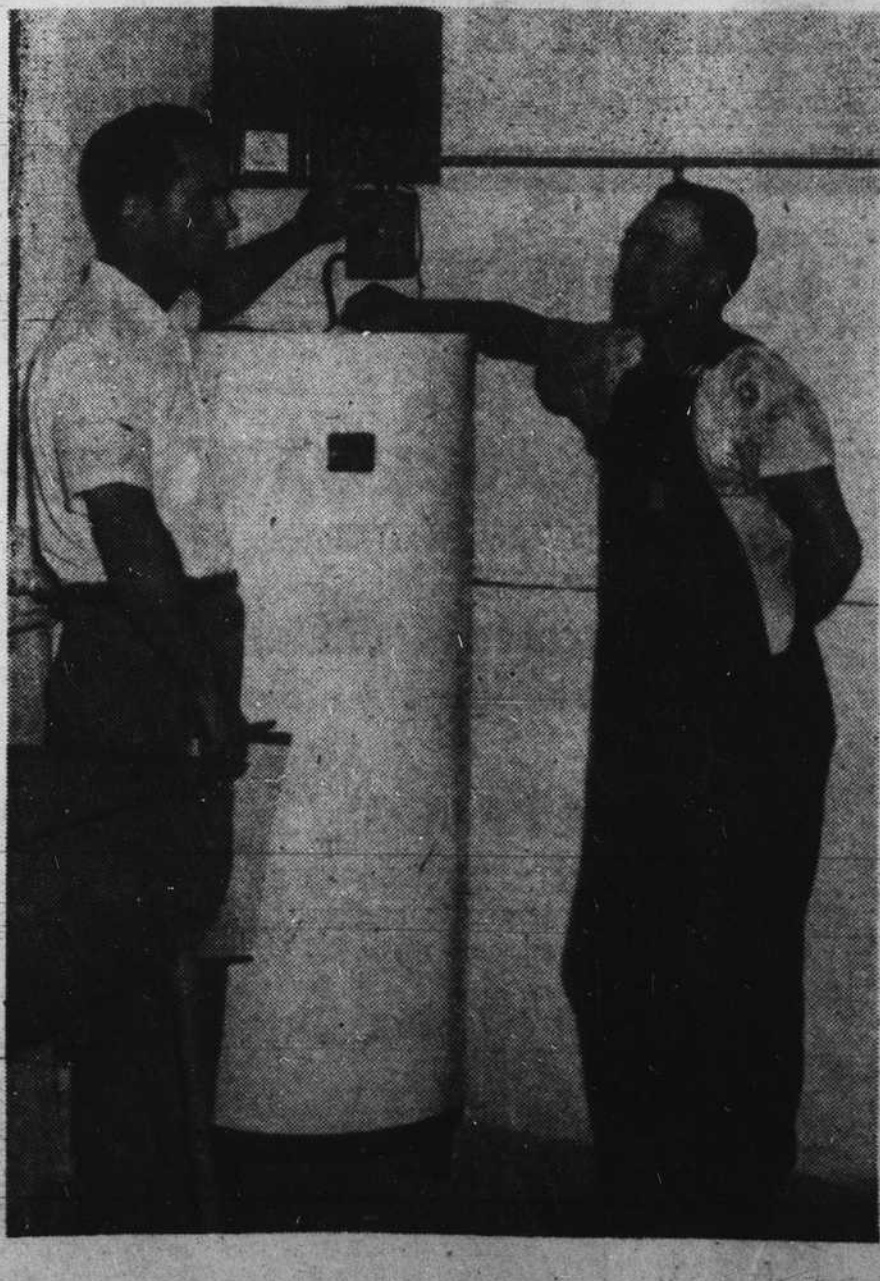
The picture at left. Vance Martin, REA engineer, discusses electrical installation with Lloyd Hall.
