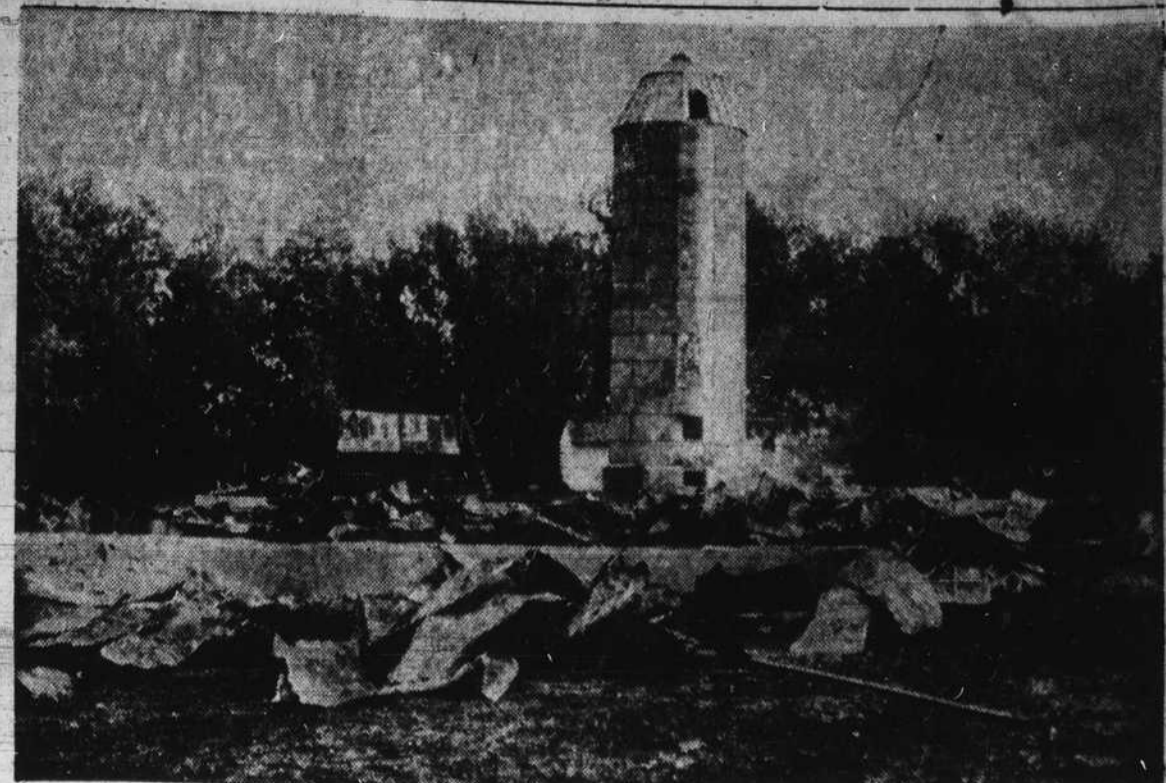
WILL SUITT'S BARN—AFTER THE STORM
