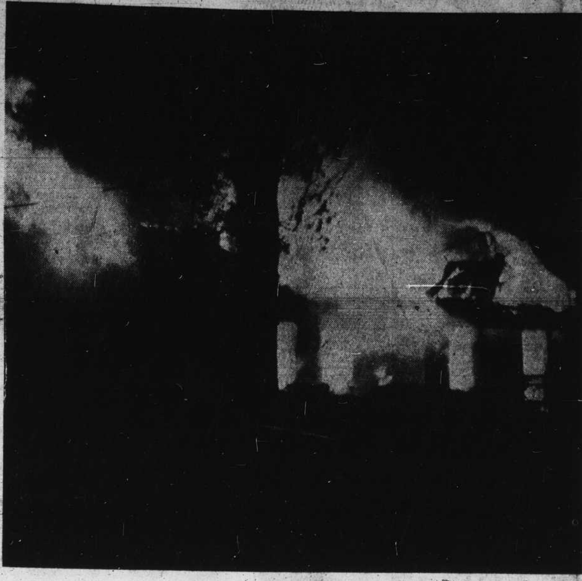
Fire destroys 6-room home of Tommy Roberts family
