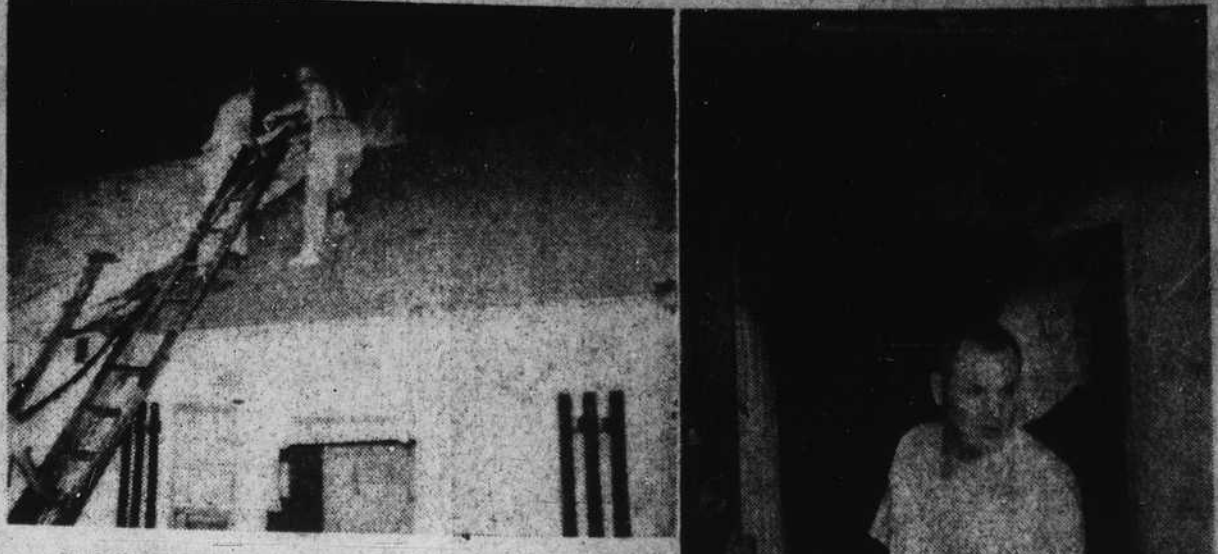
THREE TIMES AND OUT —Hillsboro firemen answered three calls to the Paul Roberts' home on Old Highway 86, three miles south of town Monday night to extinguish fires of undetermined origin. The fire apparently started in the wall of a downstairs closet and was confined largely to that area, the attic and between-the-walls smoldering.
