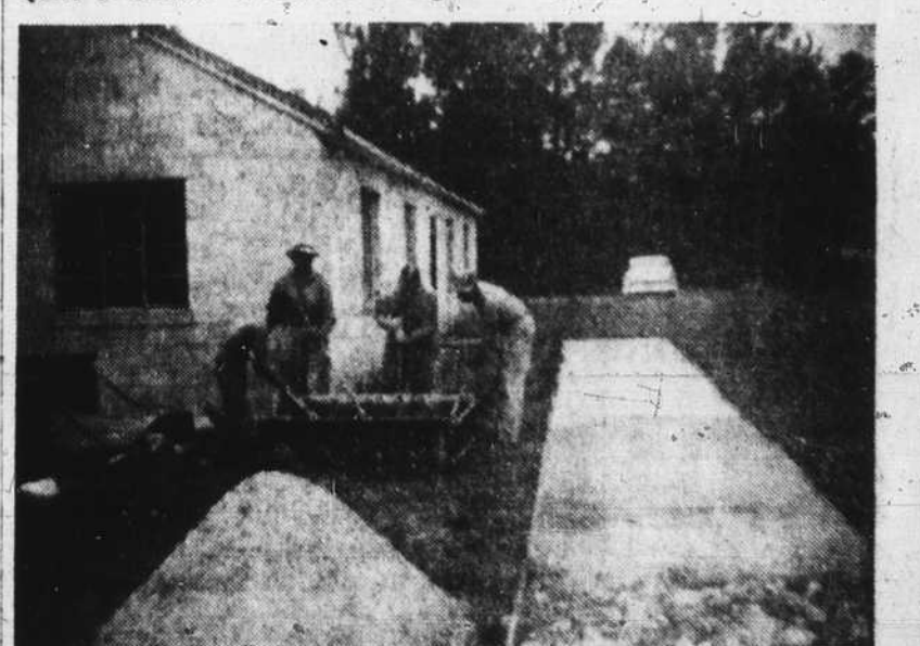
community members laying new walk for Caldwell Community Building.
