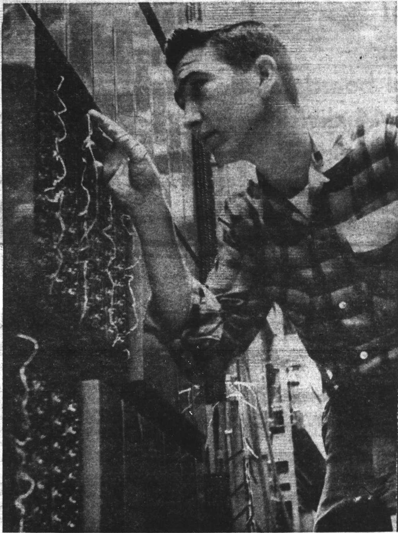
ALL SET FOR BIG SWITCH-OVER—Vernon Ray Fields of the Automatic Electric Company's installation crew shows what will be done in the Chapel Hill Telephone exchange to bring about the switch-over to the all-numerical calling system at 2:01 a.m. one month from today, Jan. 15, 1961. By simply pulling out the "blocks" linked by strings in the bays of equipment the exchange will automatically be switched in to new seven-digit set-up. (See stories on Page 4.) News Photo
