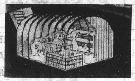
FAMILY UNDERGROUND SHELTER M-14-A-Installs 2 feet below ground level, assures considerable protection against blast as well as fallout. 116 square feet of livable space (for 10 people) -can be lengthened in sections of 20 sq. feet to accommodate 3 or more families. Complete with blower and ventilator.
