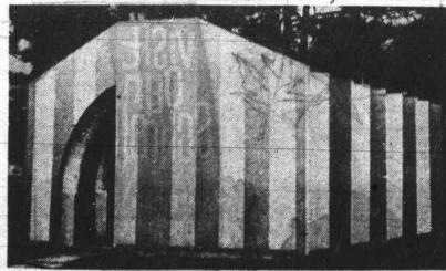
FAMILY "ABOVE GROUNND" SHELTER M-7-Designed for low cost installation on simple concrete slab with 2 feet of earth or sand coverage. Protection for 7 people (72 sq. feet)-can be lengthened in 15 sq. foot sections to accomodate 2 or more families. Complete with blower and ventilator.
