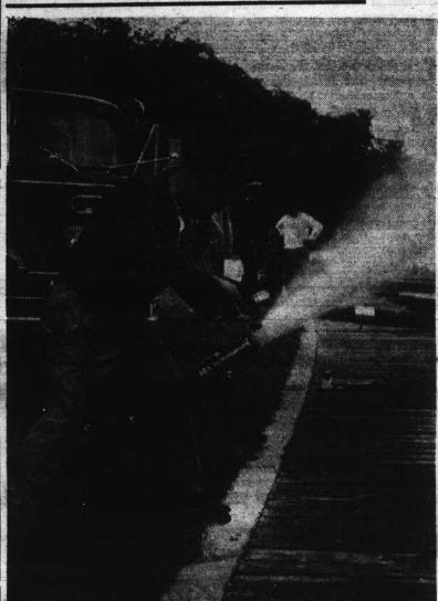
MEASURES UP—Patrick Murphy of the State Fire Insurance Rating Bureau in Raleigh meters the 1,000 gallons-a-minute water flow through a hose from Chapel Hill's new \$20,500 pumper fire truck as the vehicle was successfully passed on a required underwriters' standards in tests held at University Lake last Thursday.
