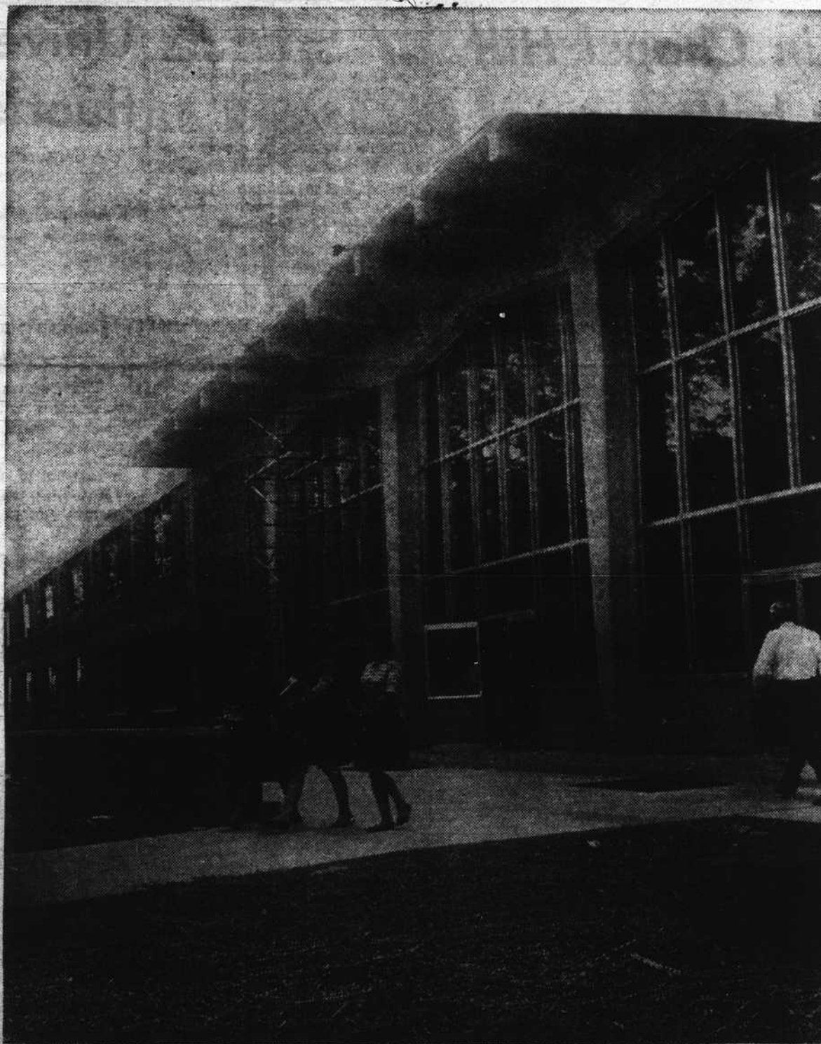
NEW HIGH FOR ORANGE — Even as workmen labored on the final stages of construction, pupils attended their first day of classes in the new million-dollar Orange High School north of Hillsboro on Monday. Above, the entrance to the high, vaulted foyer of the auditorium wing is seen, with one of two classroom wings extending into the background at the left.
