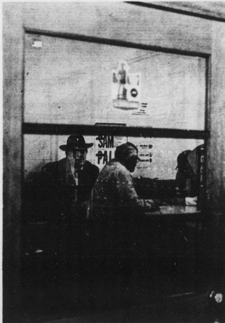
The Postal Robber, apparently entered through this door at the counter after knocking out the center glass and unlocking the door. The glass was replaced early Friday morning and business resumed as usual.
