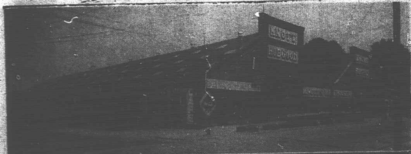
KNOTT'S WAREHOUSE No. 1
