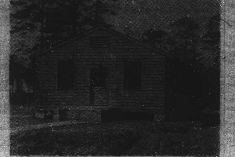
NEW SEVEN PINES CLUB BUILDING
