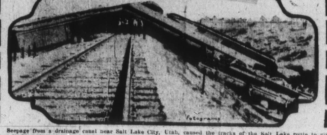
Seepage from a drainage canal near Salt Lake City, Utah, caused the tracks of the Salt Lake route to give way, ditching the crack Los Angeles flyer, killing three, and injuring many more.
