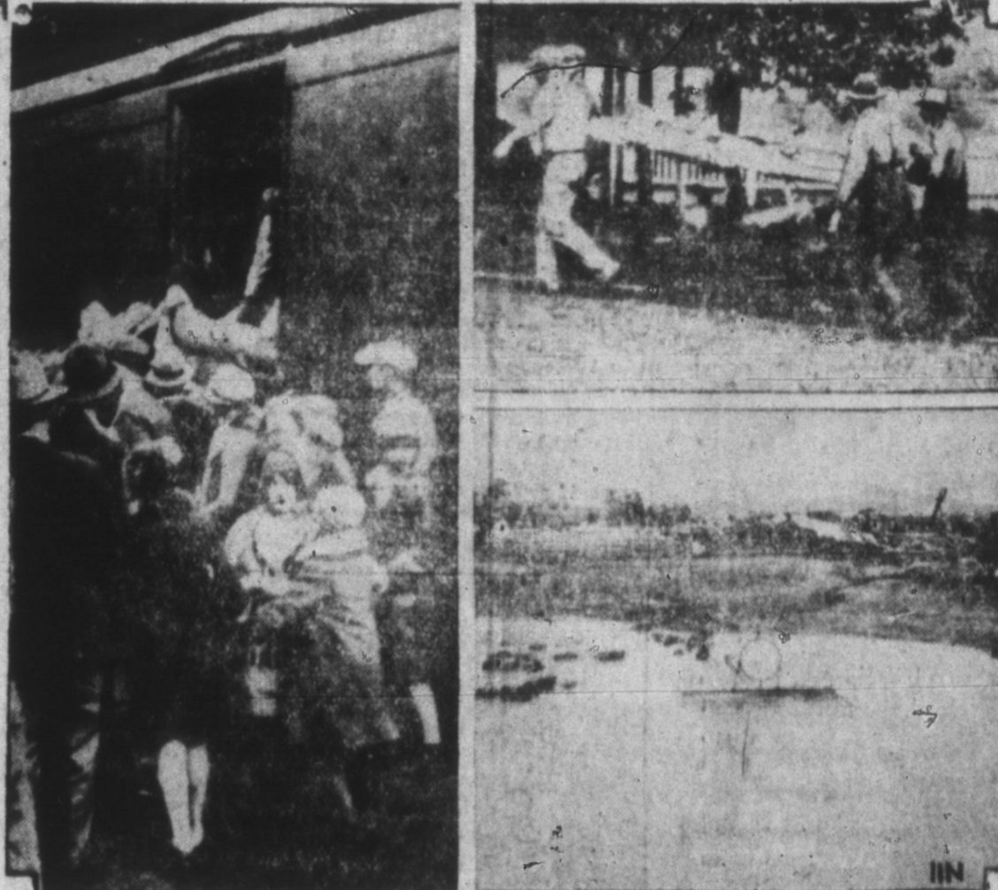
Left shows some of the 52 injured when a tornado collapsed the school at Rye Cove, Va., being placed on the train to rush them outside for medical treatment. Some of the little tots are shown, upper right, being carried from the ruins on stretchers by many of the willing volunteers who rushed to their aid. One of the remarkable stories told by survivors is illustrated below, right. Principal A. S. Noblin of the school was outside the building and saw the wind approaching. He was picked up bodily and thrown 75 feet into the pond shown in the foreground. The ruins of the school may be seen in the rear of the pond.
