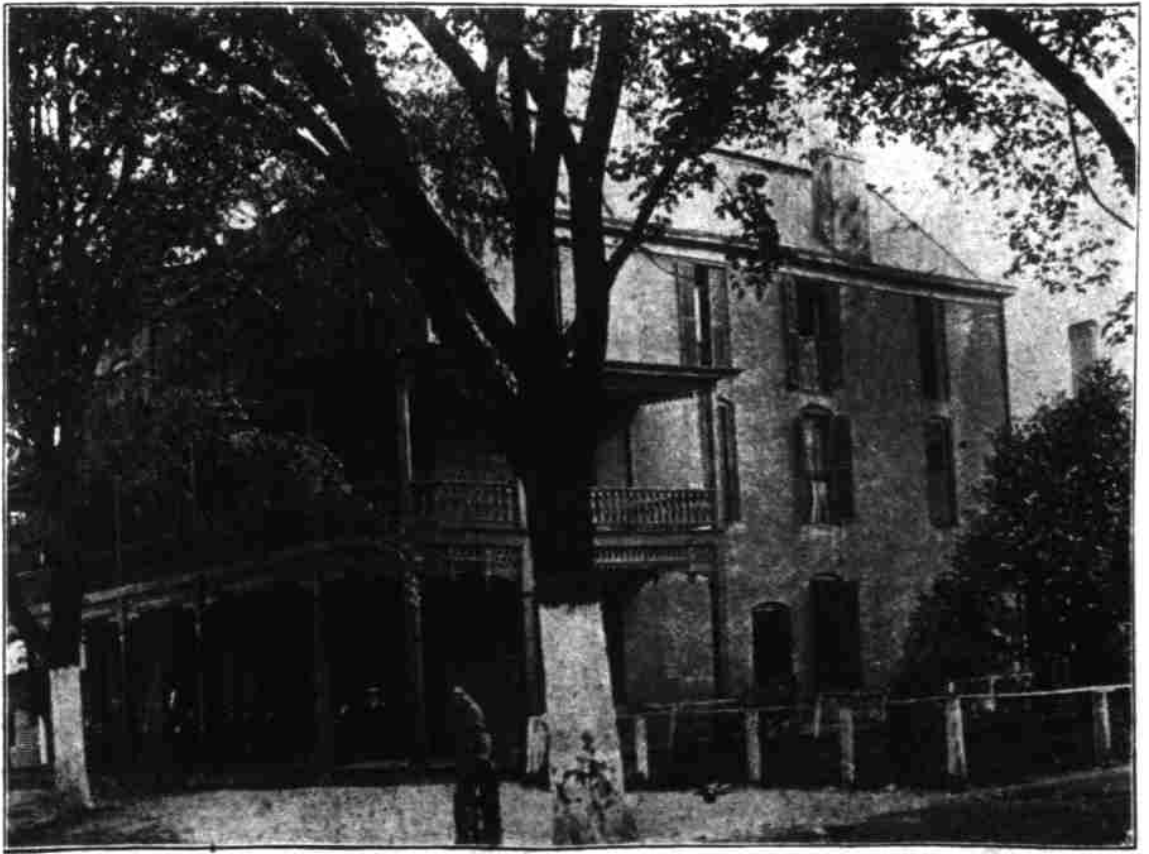
The Falls House, Gastonia, Built Thirty Years Ago and Bought Yesterday by Col. C. B. Armstrong and Mr. R. B. Babington. It is to give way to a modern hotel in the near future.
