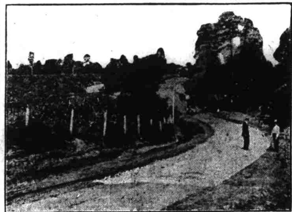
Laying First Course, Poplar Springs Road, Meridian, Mississippi.
