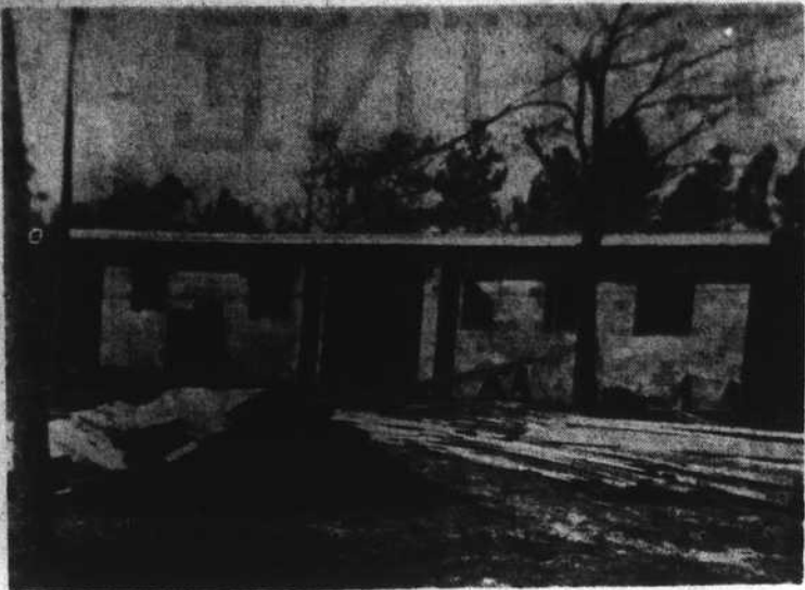
DREAM REALIZED—Members of the Scott's Store Home Demonstration club and the Herring's Store Lions club realized a dream this month when the community building, shown above, was opened. The clubs have long wanted a meeting place of their own, and in the fall of 1953 began work on the building.
