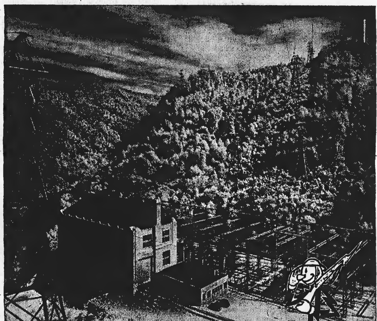
The Waterville hydro-electric development — built in keeping with our company's policy to provide, in advance of demand, an adequate source of dependable power.
