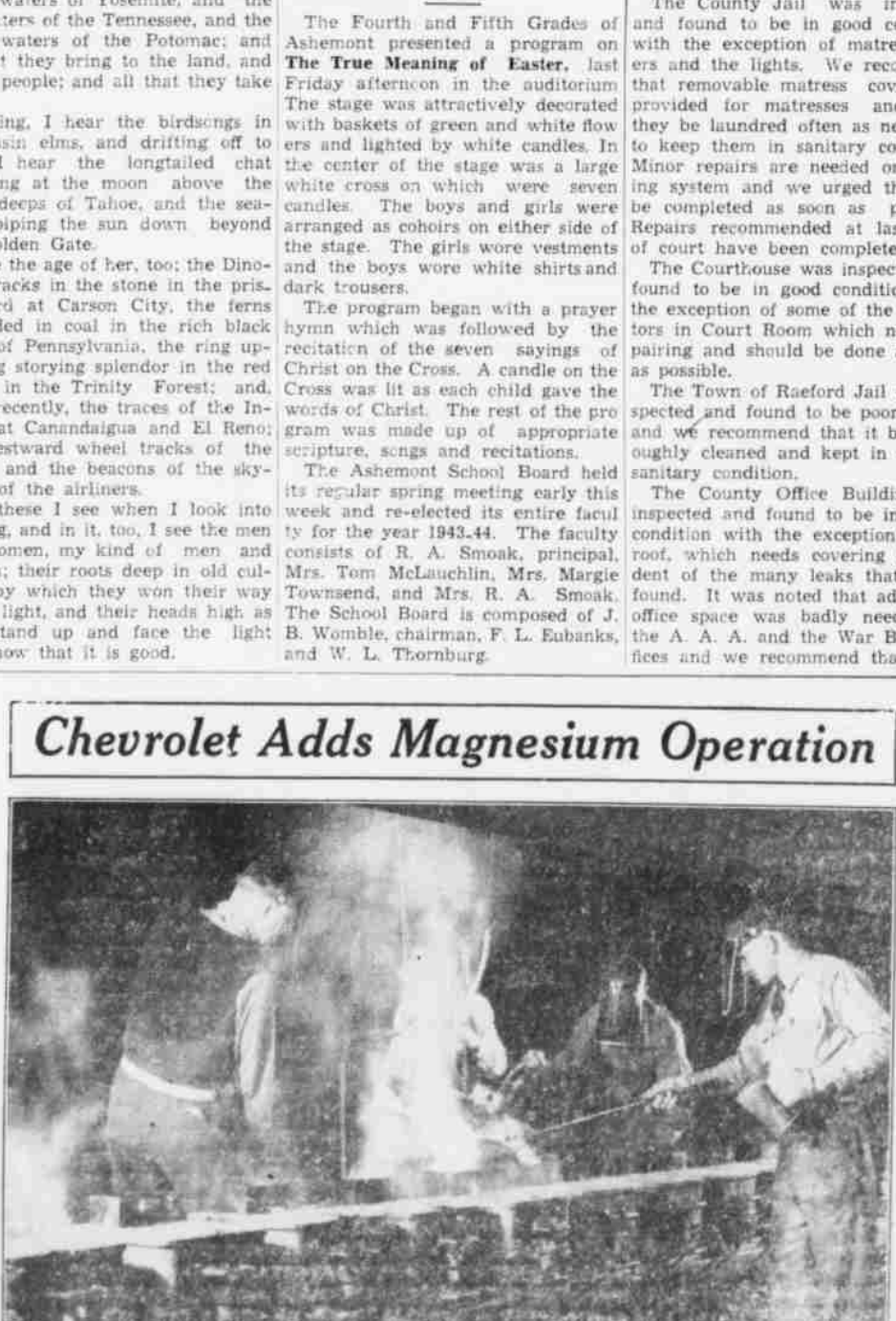
Production pouring of magnesium castings in a division of the Chevrolet Grey Iron Foundry in Michigan is now an accomplished fact, adding a considerable new output of these vital aircraft engine parts to America's war production program. Shown above pouring this highly volatile new metal are workers in the Chevrolet plant.
