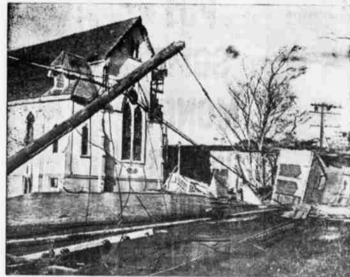
The big blow twisted the steeple off this Massachusetts church and toppled it into the street across the electric wires. Another headache for hard-working linemen!
