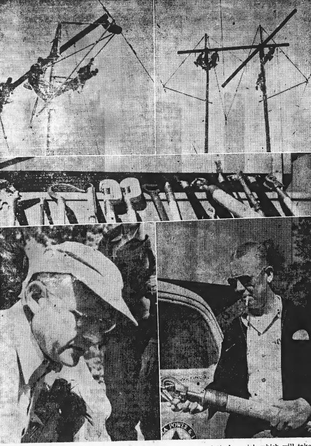
disconnecting the "hot line" from and here is being swung across to crew, holding a grasping hot an insulator. Notice how the line to the adjoining pole. has been held safely away from Center shows some of the many wire, the clamps may be tightenthe working men by two "hot sticks employed in the new me- ed like a fist by turning the other sticks" lashed to a pole. If a man the high voltage line, an arc "heads" are used and the man might leap to him from the con-
