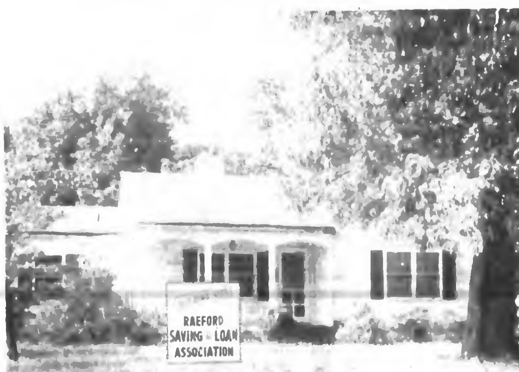
STE - The building site for the new Raeford Savings and Loan Association is at 113 Campus St. This dwelling house will be moved away to make room for the new building.
