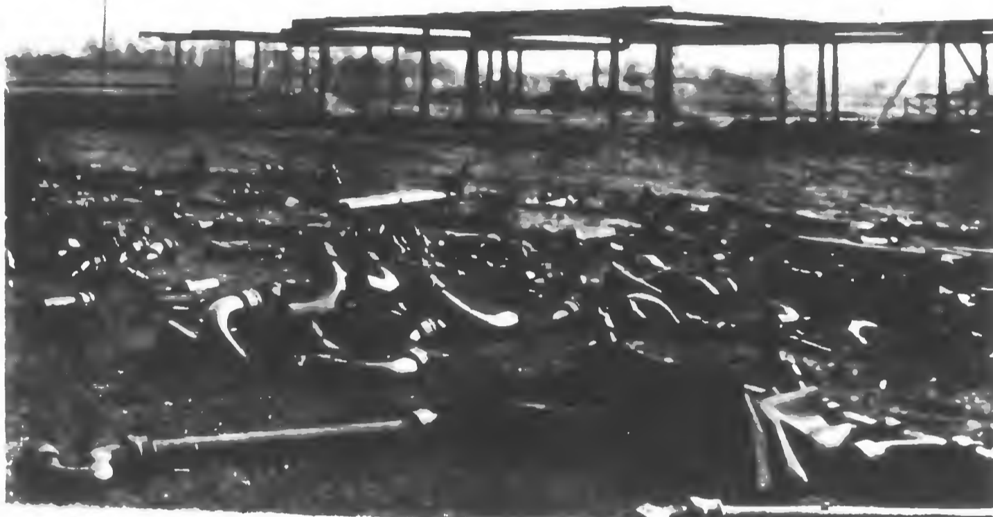
Water And Sewer Pipes Await Installation At New School
