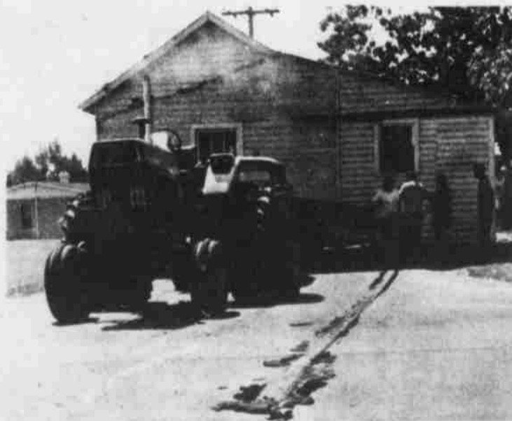
WHAT TO DO NOW? - L. C. Cunningham and Foster McBryde were moving this house for Mrs. Ruthie Davis, from Oakwood Avenue to her lot on Turnpike Road. They ran into complications at the intersection of Central Avenue and Jackson Street. The house was left in the middle of Jackson Street until a solution could be found. At last report, the house still had not been moved.
