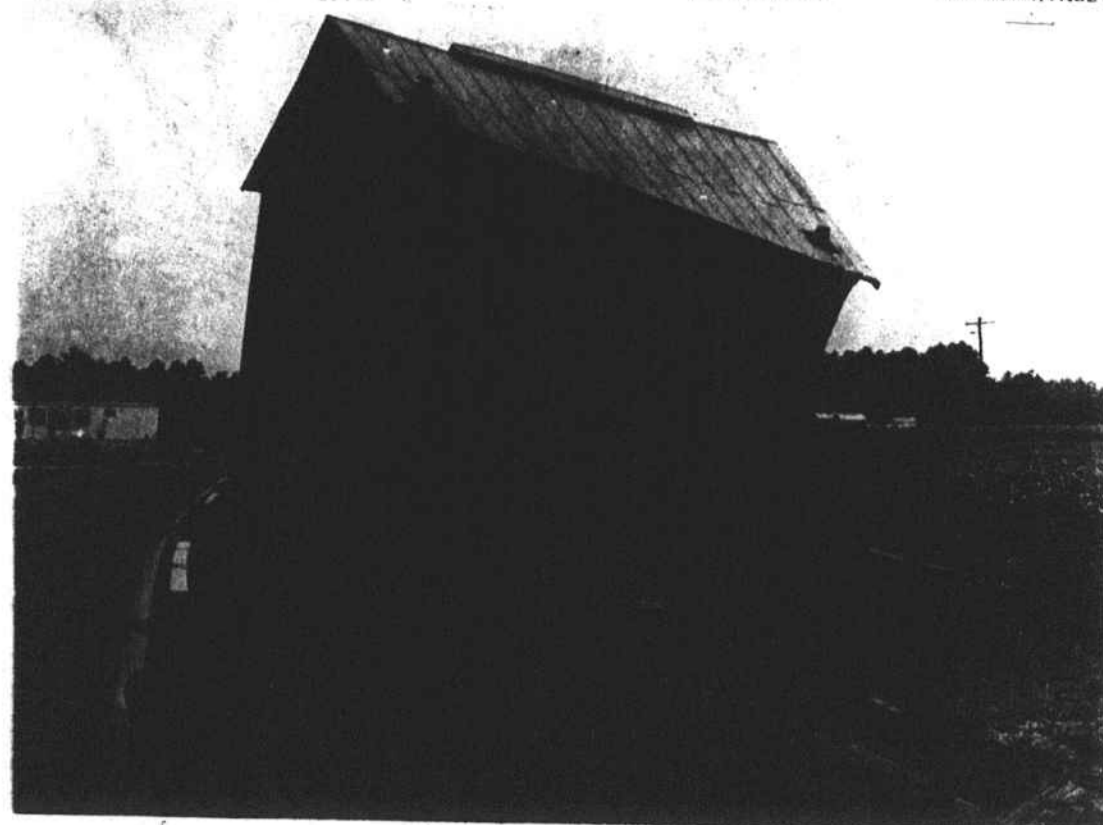
TOBACCO (BARN) ROAD - The barn was being moved from the McGougan farm in the Sandy Grove section to the Joe Scott farm in the Gold Hill section when the foundation gave way on one side causing it to slide partly off the truck less than 100 yards from its destination. The mishap occurred Saturday morning.
