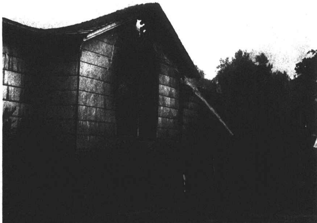
HOLLOW SHELL - The inside of the home was completely destroyed and only part of the outside walls remained when firemen from Raeford and North Raeford fire departments put out the fire at the Hunter Carroll home off the Aberdeen highway last Thursday.
