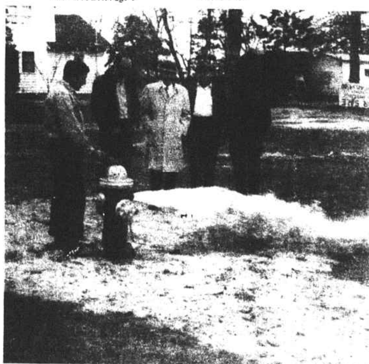
WATER - James Dobbins, contractor, turns on the water for the new Rockfish Community Water System as the board of directors make a final inspection and accept the system. Show left to right are Dobbins, Lacy Koonce, engineer, and board members, Herman Koonce, Tommy McInnis and Burnice B. Bostic, chairman of the board. Not present are Ralph Barnhart, Linda J. Gaddis, Donald Wood and K.P. Ritter.
