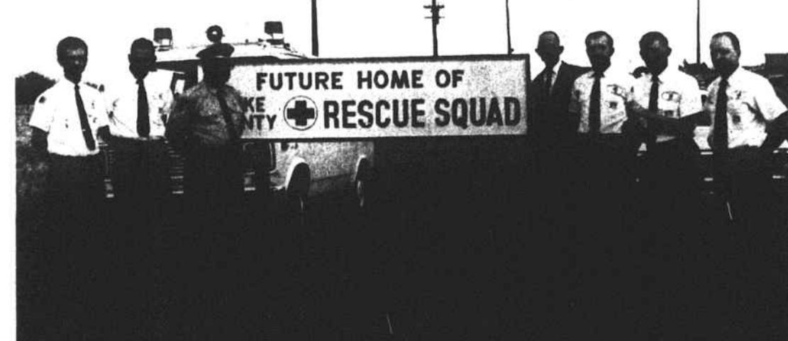
RESCUE GROUND BREAKING - Ceremonies to begin the construction of the new home of Hoke County Rescue Squad, Inc. are shown above with William T. Parker digging first foundation spade full. (Left to right) squad members Eric Allen, Charles Tew, city policeman Leonard Wiggins; chairman county commissioners, T.C. Jones and squad members Winfred Walters, William T. Parker, Jim Wade.
