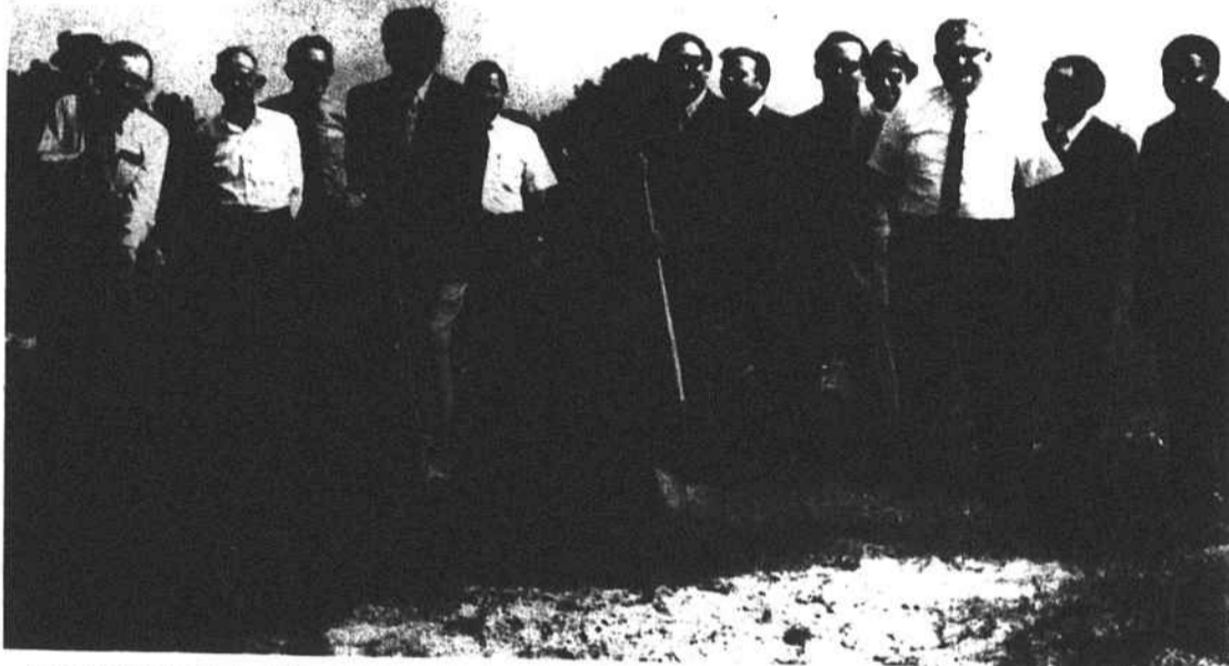
GROUNDBREAKING - Officials and guests man shovels at groundbreaking ceremonies held Monday by the Hillcrest-Scurlock Community Water System, Inc. From left are Smith McInnis, water system president; E.E. Smith, clerk of court; T.C. Jones, chairman, county commissioners; M.R. Mills, county sanitarian; Jimmy Morrissy, system vice-president (with shovel); Bobby Conoly, system director; James T. Johnson, state FHA director (with shovel); Palmer Willcox, city attorney; C.D. Bounds, president of Chamber of Commerce; D.B. McFadyen, water system director; Tommy Macko, water system director; Jake Vinson, county FHA supervisor; the Rev. Milton Williams, system member.
