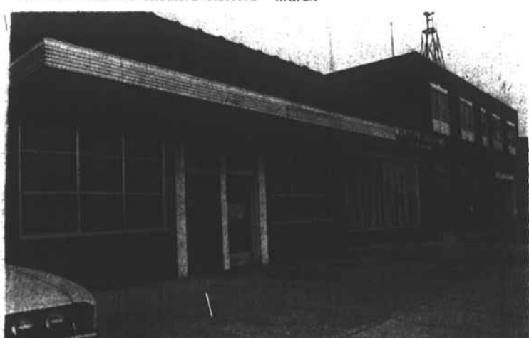
CITY APPROVES PURCHASE - The City Council Monday agreed to purchase this single - story section of City Hall. The two - story section houses the Water Department, garage, Police Department and Fire Department and is owned by the city. The one - story section, houses offices occupied by the city manager and the Teen Center. It has been occupied on a lease - purchase agreement and is owned by Thomas, Snead and McNeill.
