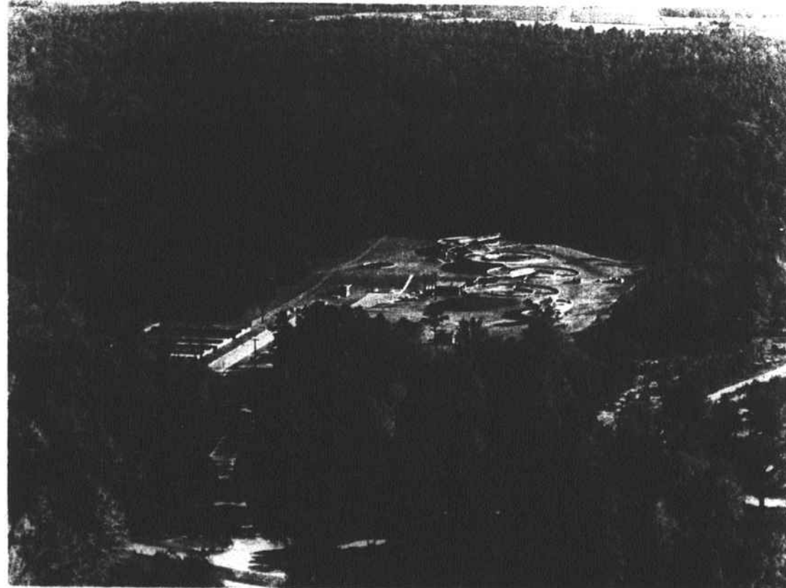
CITY REIMBURSED—Pictured is the city's sewage treatment plant, one project on which the city is to receive federal grant of $119,800 in reimbursement funds. The Environmental Protection Agency made the funds available after Congress ruled that federal funds should be available for 50 percent of the total cost of such projects instead of the 30 percent rule in effect when the project was begun. Other projects on which the city applied for reimbursement funds include the 1969 enlargement of the plant by 1.5 million gallons per day, and the 1971 construction of interceptor sewer lines used mainly to supply water and sewer service to Knit-Away, Inc.
