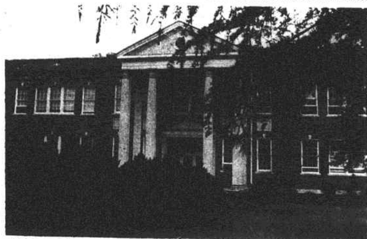
NOT SUITABLE - A state survey team reports, "Most of the buildings at Raeford Elementary School are nonfire-resistant; the total facility is not worthy of extensive renovations due to the limited site and to its poor condition for educational purposes." The state Division of School Planning survey report recommends two options for the Hoke County School system. Both options include discontinuing use of Raeford Elementary building as a school (N-J Photo)
