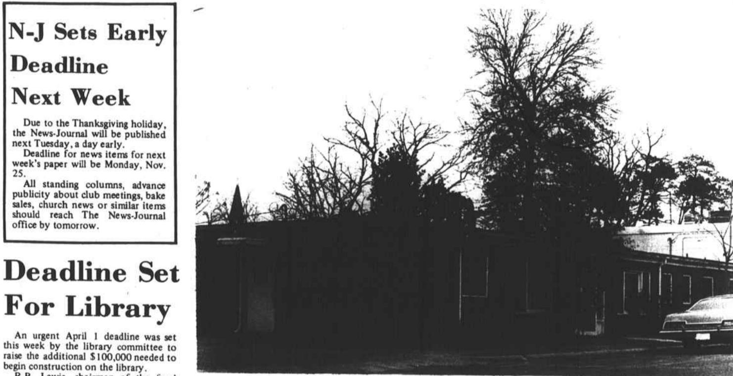
REST HOME... will be doubled in expansion program.
