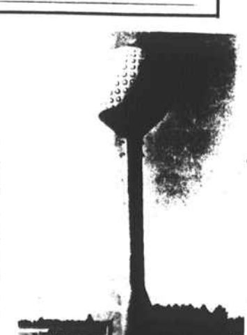
Largest golf ball in the world? Actually, the water tank supplying our completed central system.
