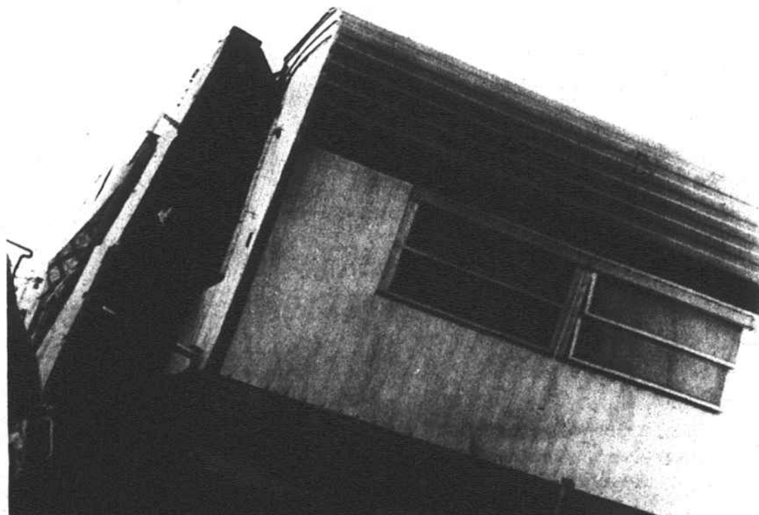
DAMAGED - While not demolished, this trailer at West Hoke was hard hit by wall of the neighboring mobile home.
