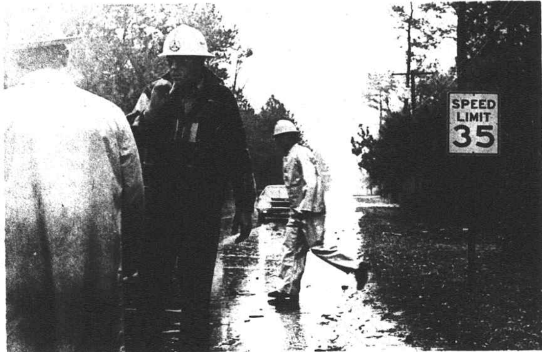
REPAIR - CP&L workers remove downed power lines from North Fulton Street.
