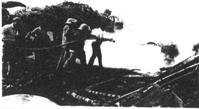
FIRE PUT OUT -About nineteen firemen responded Thursday afternoon at the Raeford Salvage Yard when thick black smoke attracted a large crowd of onlookers. Fire Chief Crawford Thomas said a cutting torch had ignited fuel oil inside a transformer. The blaze was quickly put out with no injuries. (Photo by Ken MacDonald).
