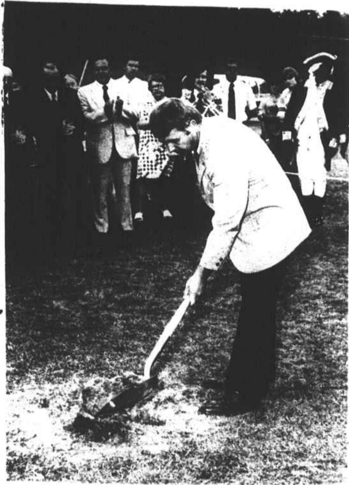
COUNCILMAN —Benny McLeod, city councilman, stepped up with a shovel at the groundbreaking to turn the beginning of the library as the crowd applauds.
