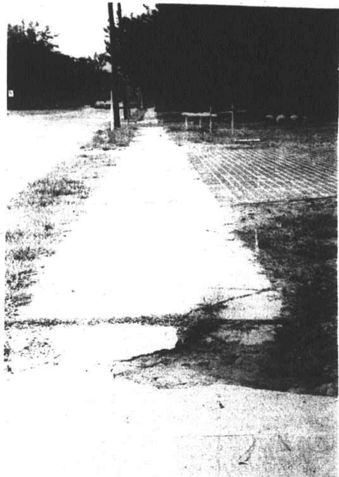
SIDEWALK DIG - City manager Robert Drumwright got in his digs, too, last week as the controversy over the appearance of the sidewalk in front of the new library building resulted in the arrest of a construction superintendent for destroying city property, or digging up sidewalk.
