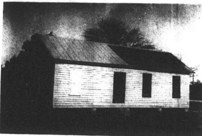
SCOUTS' HOME -- Z.V. Pate Inc. of Laurel Hill donated this house to Boy Scout Troop 434. If the Scouts can interest community groups in helping furnish their new meeting place, they hope to be able to move in by next February.
