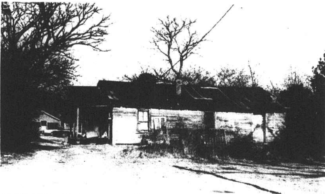
TARGET AREA -- This is one of scores of dilapidated and sub-standard homes in the section north of town known as Jones Hill. The county plans to spend $87,000 in federal funds to repair homes in Jones Hill, Cameron Heights and Silver City.
