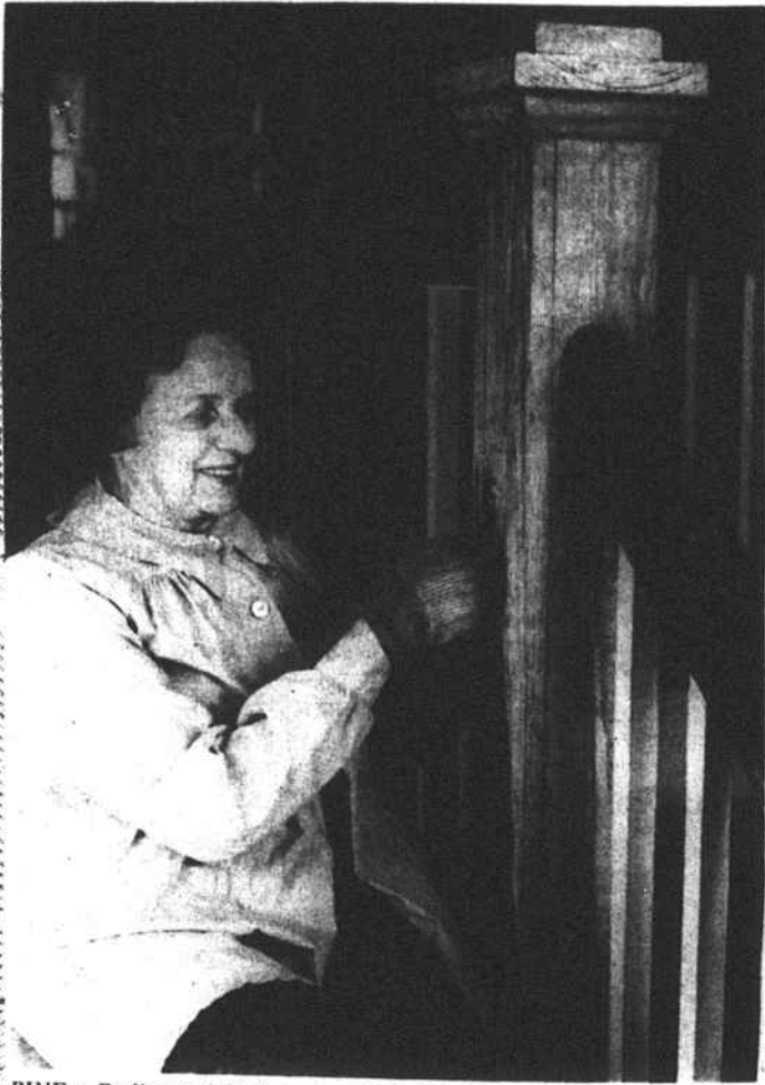
PINE -- Rediscovering the natural beauty of a heart of pine baluster with pine balusters is Mamie Gatlin. Mrs. Gatlin has spent about three weeks in her home scraping off a 40 year-old layer of mahogany paint. When she finishes scraping the paint off and smoothing with a special liquid sand paper, Mrs. Gatlin plans to seal the wood with tung oil. The project has been carried out in consultation with the extension home economics agent, who is available to county residents for free remodeling advice. (Photo by S.H. Aplin)
