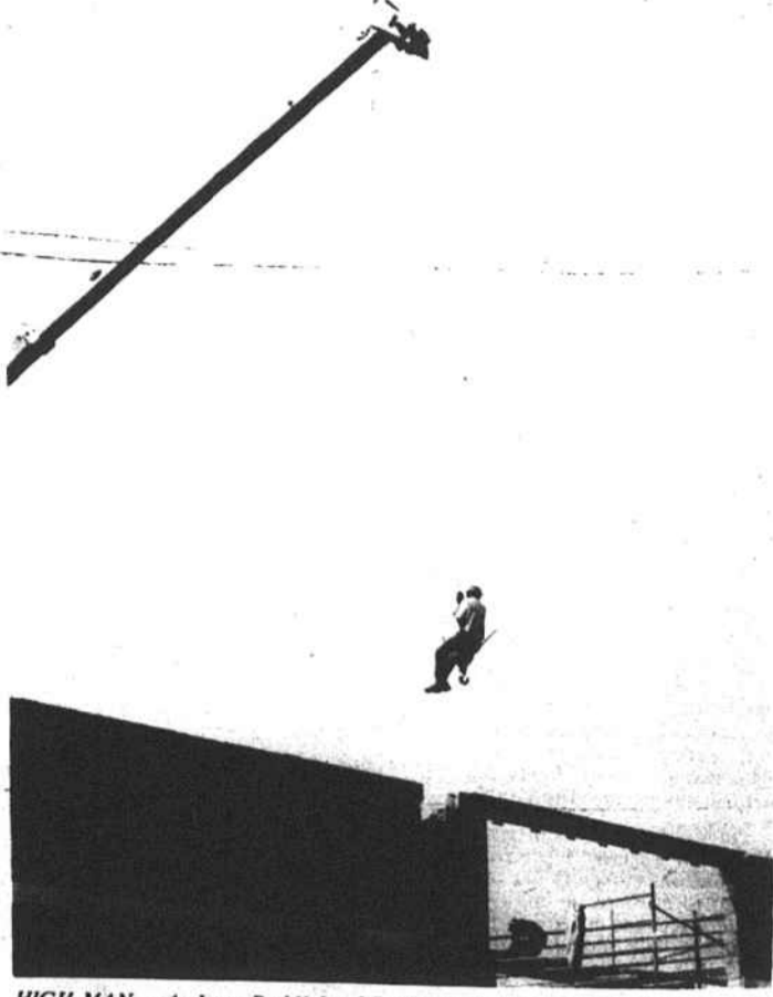
HIGH MAN - Andrew Reddick of Rockingham rides a derrick ball over the new office building of The Bank of Raeford in downtown Raeford. He was about 30 feet above ground when this picture was taken Friday afternoon.
