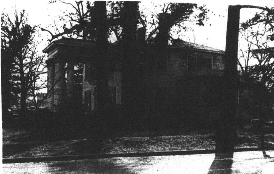
The Austin home Monday morning after Sunday's fire...Some damage shows on the roof right of center.
