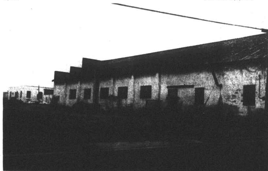
Part of land county is buying for more office space. The view is looking southwest. The picture was taken from the front of the sheriff's department building. [Staff photo by Bill Lindau.]
