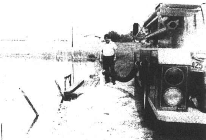
Fire Chief Johnny Baker at dry hydrant [white] and pumper truck. Truck's black hose will be connected to the hydrant and truck and water pumped into fire department tanker truck.
