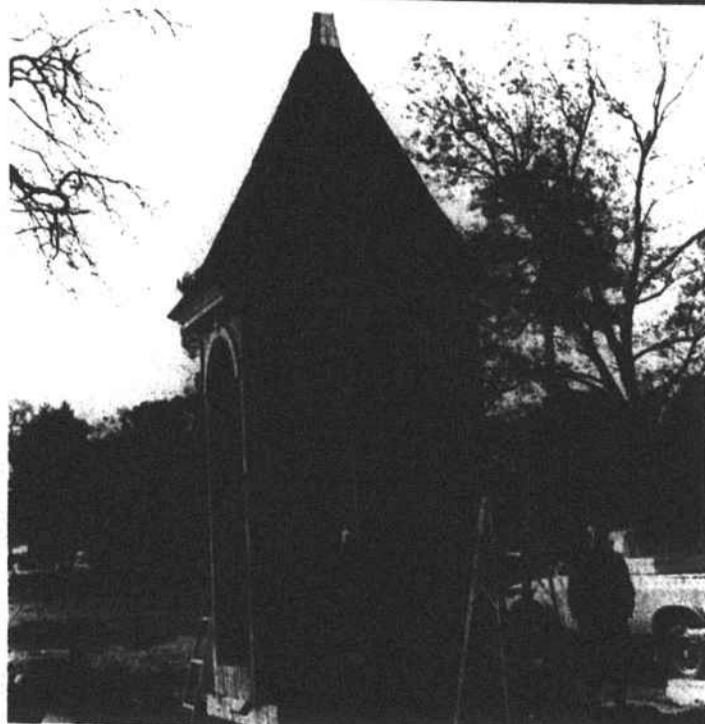
NEW HOME -- The old bell and steeple of First Baptist Church of Raeford were being set up in the area behind the old and new sanctuary buildings last week for continued life. They were taken from the old frame sanctuary building as the new building was being completed. The belfry's original exterior is being replaced by new material. The old building's life also is being continued, for educational programs.
