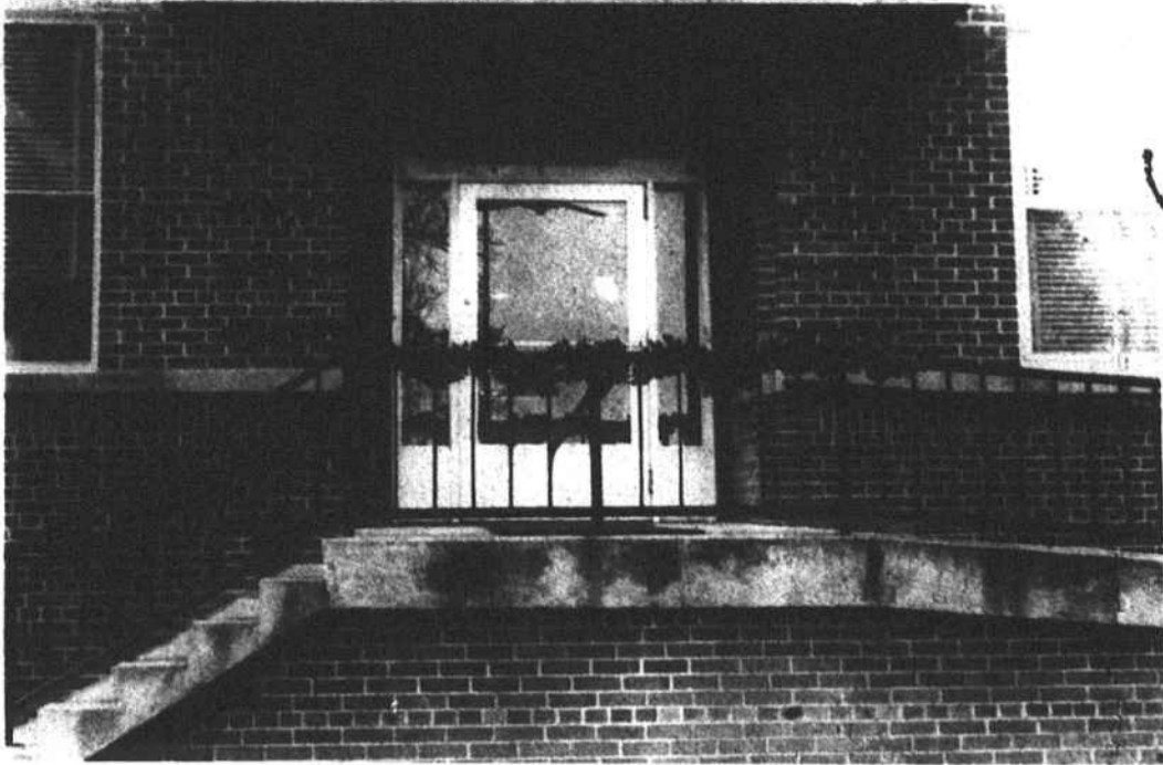
Decorated railing at main entrance of McCain Hospital.
