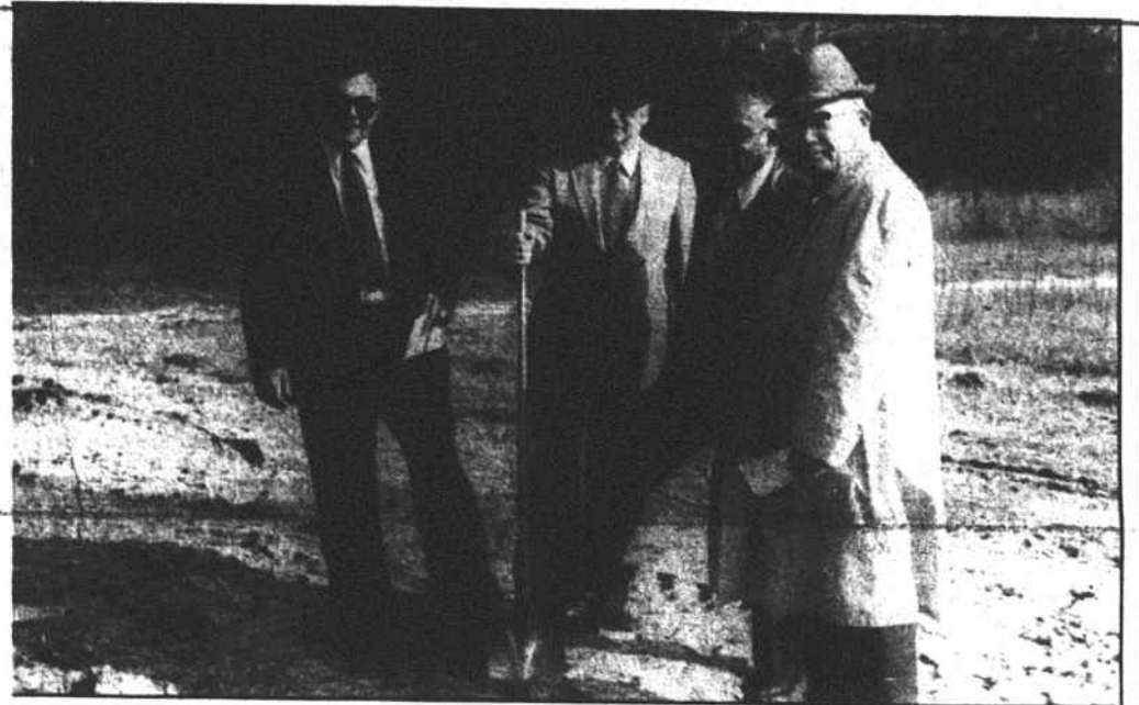
NEW HOUSING -- Raeford Mayor John K. McNeill, Jr., broke ground formally Tuesday morning for construction of The Meadows, on North Fulton Street near U.S. 401 North. The Meadows will consist of 15 one-story brick veneer buildings containing two apartment units each, for low- and moderate-income families. L-R are Raeford Housing Authority Chairman J.H. (Buddy) Blue, Jr., McNeill, Authority Vice Chairman J.D. McAllister, and Authority member Leonard Miller. Other Authority members who attended were Betty H. Morgan, Harold E. Stone, Prince Black, and James Attaway. Other Hoke County and Raeford city officials, State Human Resources Department representative Donald Huffman, Avery Connell, who sold the property to the builder and developer -- Brown, Loving Co. of High Point -- and T.A. Loving of the firm. Loving said the project is expected to be ready for the tenants by August and excavation of the 4.5 acre site probably would start this week if the weather is favorable. The building cost will be about $1 million. Of the apartments, 16 will contain two bedrooms and the others three bedrooms. The Housing Authority will be the manager of the residences. Help from Section 8 of the U.S. Rental Assistance Program will be available to eligible tenants.
