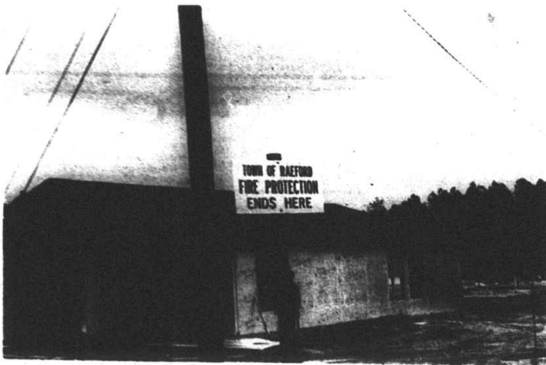
IS IT OR ISN'T IT - By the appearance of the sign the new housing project under construction is not in the Raeford Fire District. The sign, however is wrong. The area has been annexed into the city and will allow fire protection for the upcoming 30 units that are rent subsidized.
